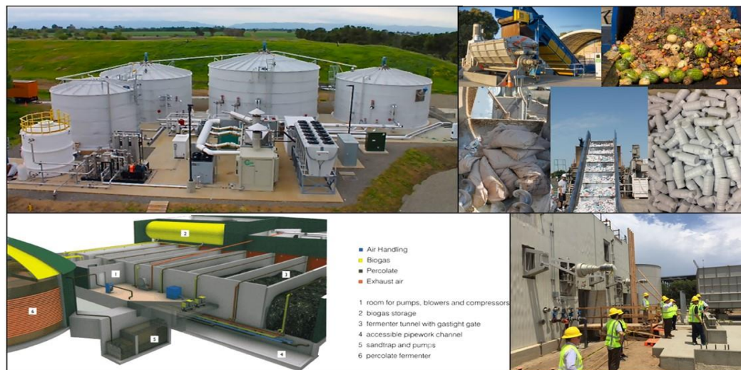
Above: Wet AD system processing food wastes on UC Davis campus. Below, Dry AD engineered by Kompoferm (Germany), and CR&R dry AD system in Perris, CA, July-2015.
